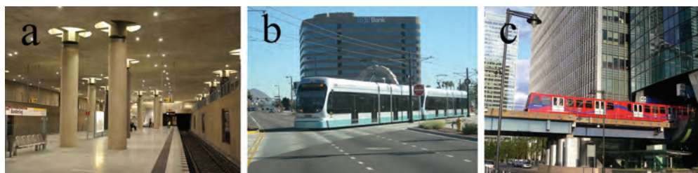
Figure 1: Position of the route: a) the underground metro tracks in Berlin, Germany (Eric Pancer), b) light rail system at ground level in Phoenix, USA (John Hall & Associates), c) light rail system above ground level (on the viaduct) in London, England (www.funini.com).
