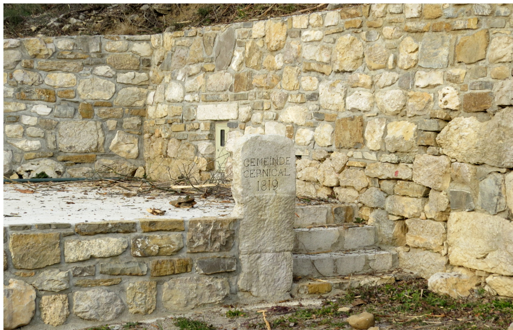
Figure 19: Relocated boundary mark in the village of Gabrovica from the time of the Franciscan land cadastral survey (photo: M. Triglav Čekada, 2024).
